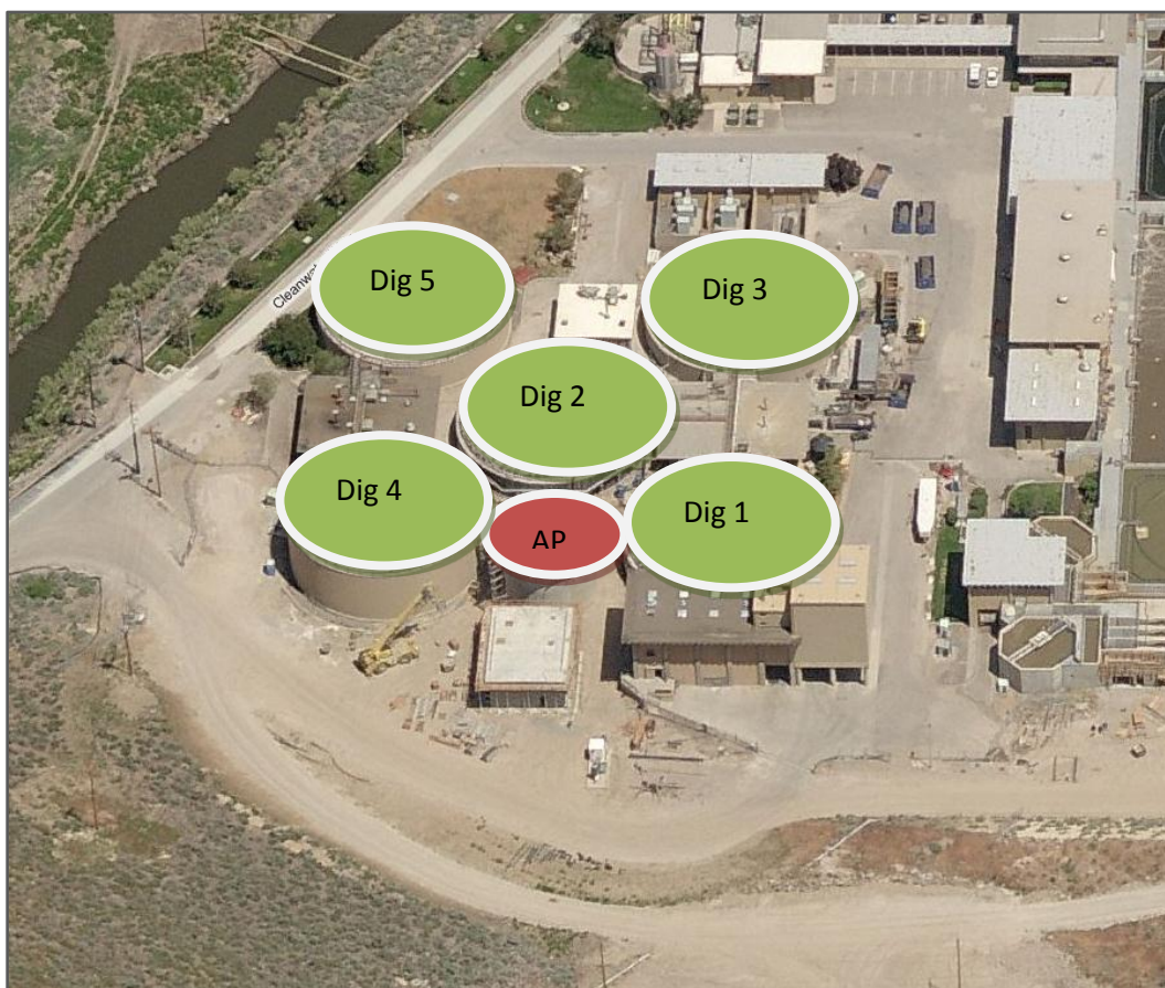
Figure 4.7. TMWRF Biosolids Digestion Facility
