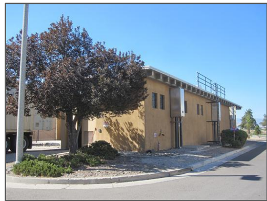
Electrical Equipment Building
