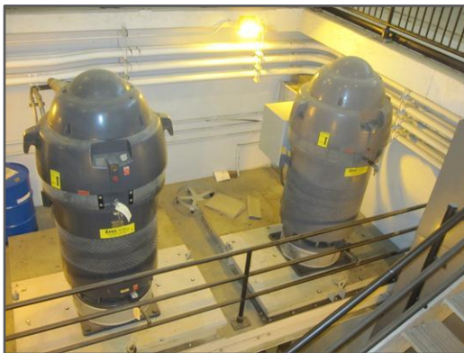
Raw sewage pumps at the Headworks Building. Pump motors (left); Pump shaft to wet well below (right).
