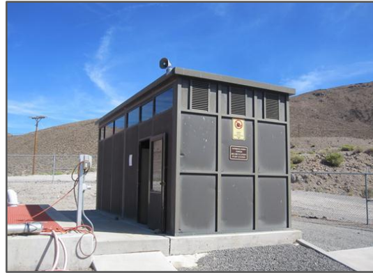
Nitrification Tower Recirculation Pump Station
