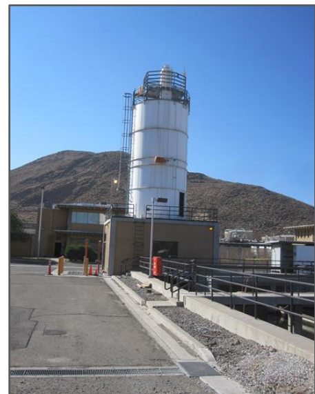
Chlorine Contact Building and basin. The storage silo was removed in 2012.
