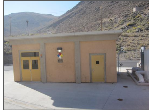
Ferric Chloride Building
