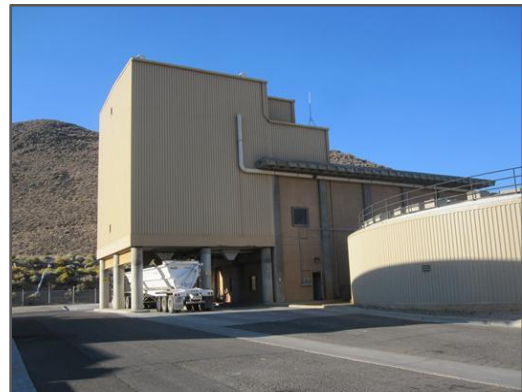
Solids Dewatering Building
