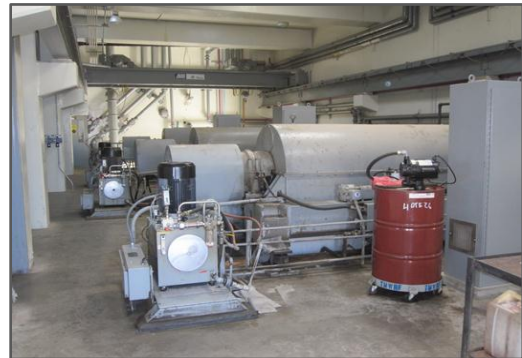
Dewatering centrifuges
